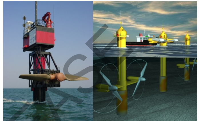
Figure 3 left: prototype „Seaflow“ at the west coast of Britain (photo: ISET) right: planned OCPP (graphic: Marine Current Turbines ) Source: Quaschnig, V. (2007): Regenerative Energiesysteme – Technologie, Berechnung, Simulation , 5. Auflage, München: Hanser-Verlag 2007
