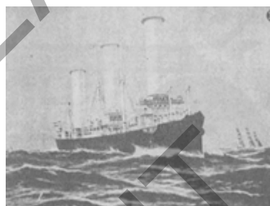
Figure 7. Anton Flettner's rotor-ship.
