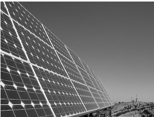
Figure 7. Solar Panels – Spain
