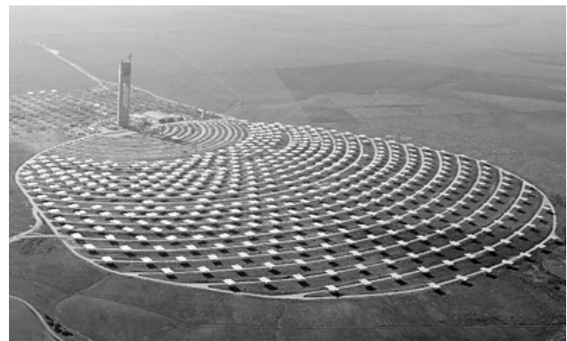
Figure 3. PS 10 power plant (bird's-eye view)
