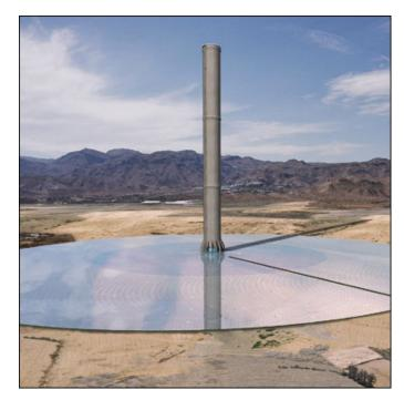
Fig. 4: solar updraft power plant
